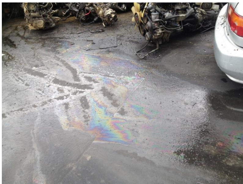
21.2 Figure 22: Substantially non-compliant worksite, oils and fuels on ground create a slip hazard
