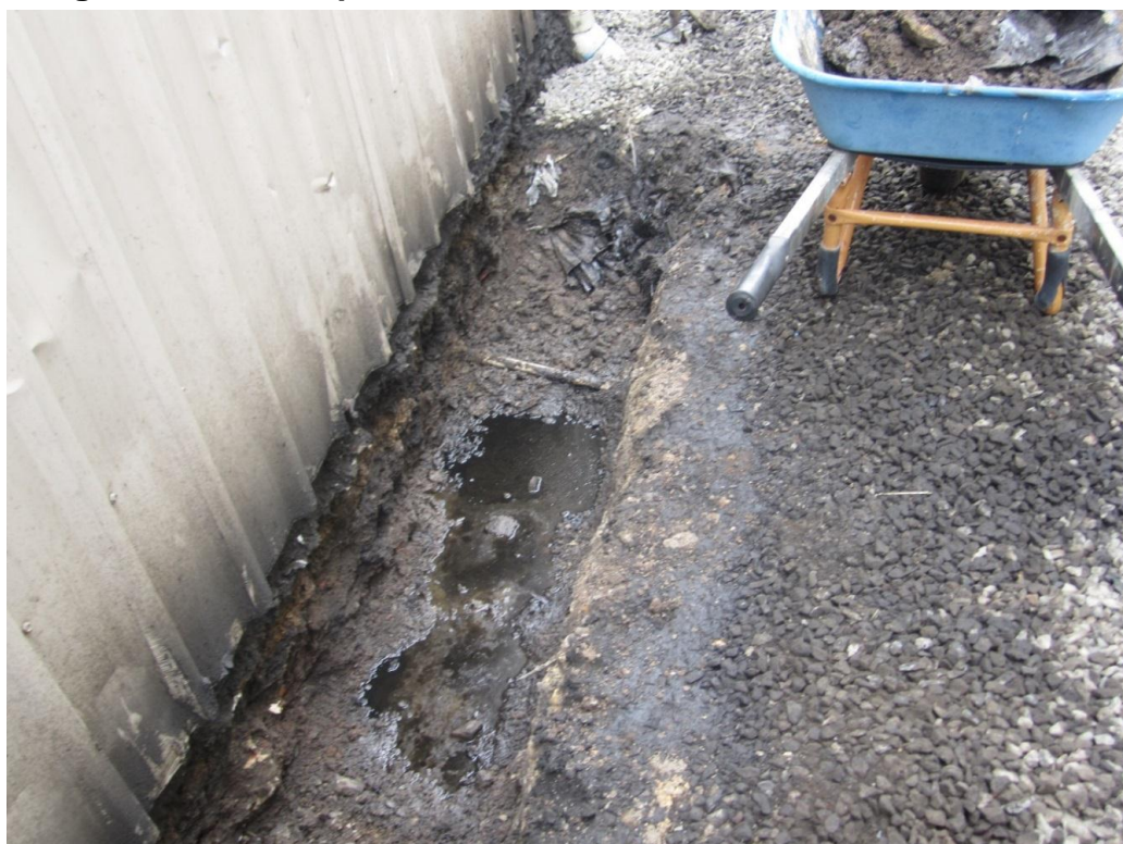
22.4 Figure 28: Completely non-compliant worksite oils, fuels and other vehicle fluids leaking into unsealed pit
